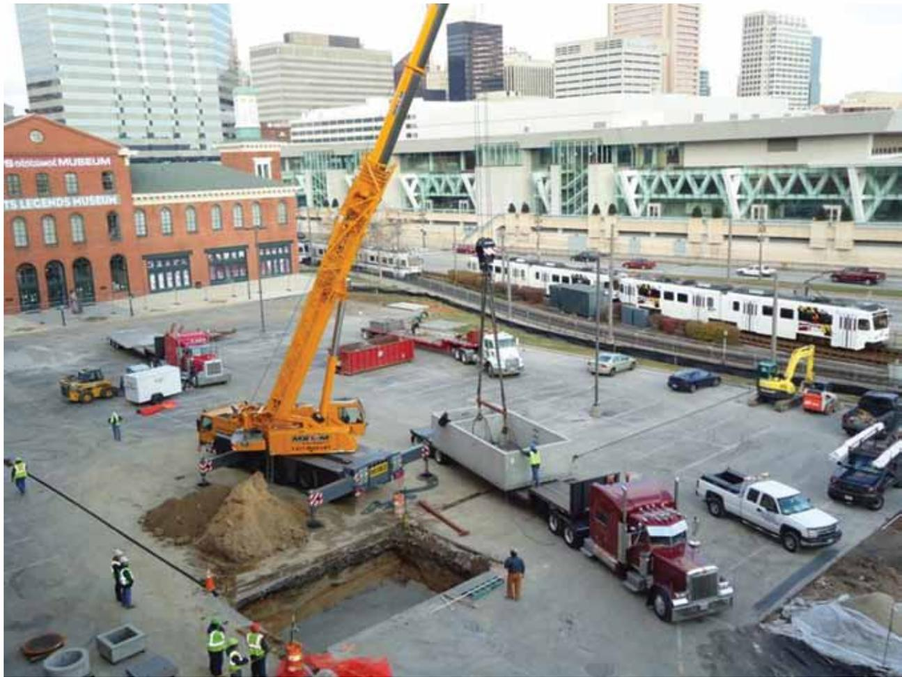
As part of the lot improvements for Pit Row at Camden Yards, the Stadium Authority installed a 7000 gallon underground reservoir to collect rain from the Warehouse roof. This stormwater management device will be pumped for irrigation and power washing, significantly reducing potable water use.
