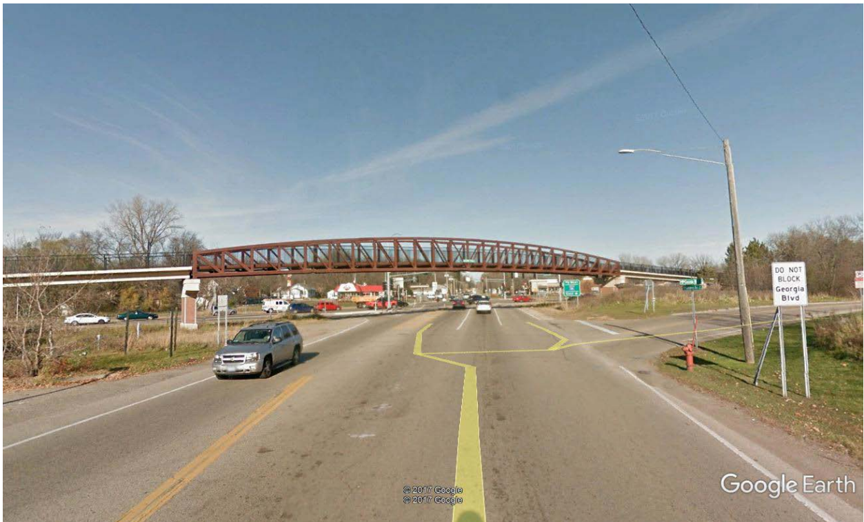
Gateway Trail Iron Bridge, Minneapolis, MN
