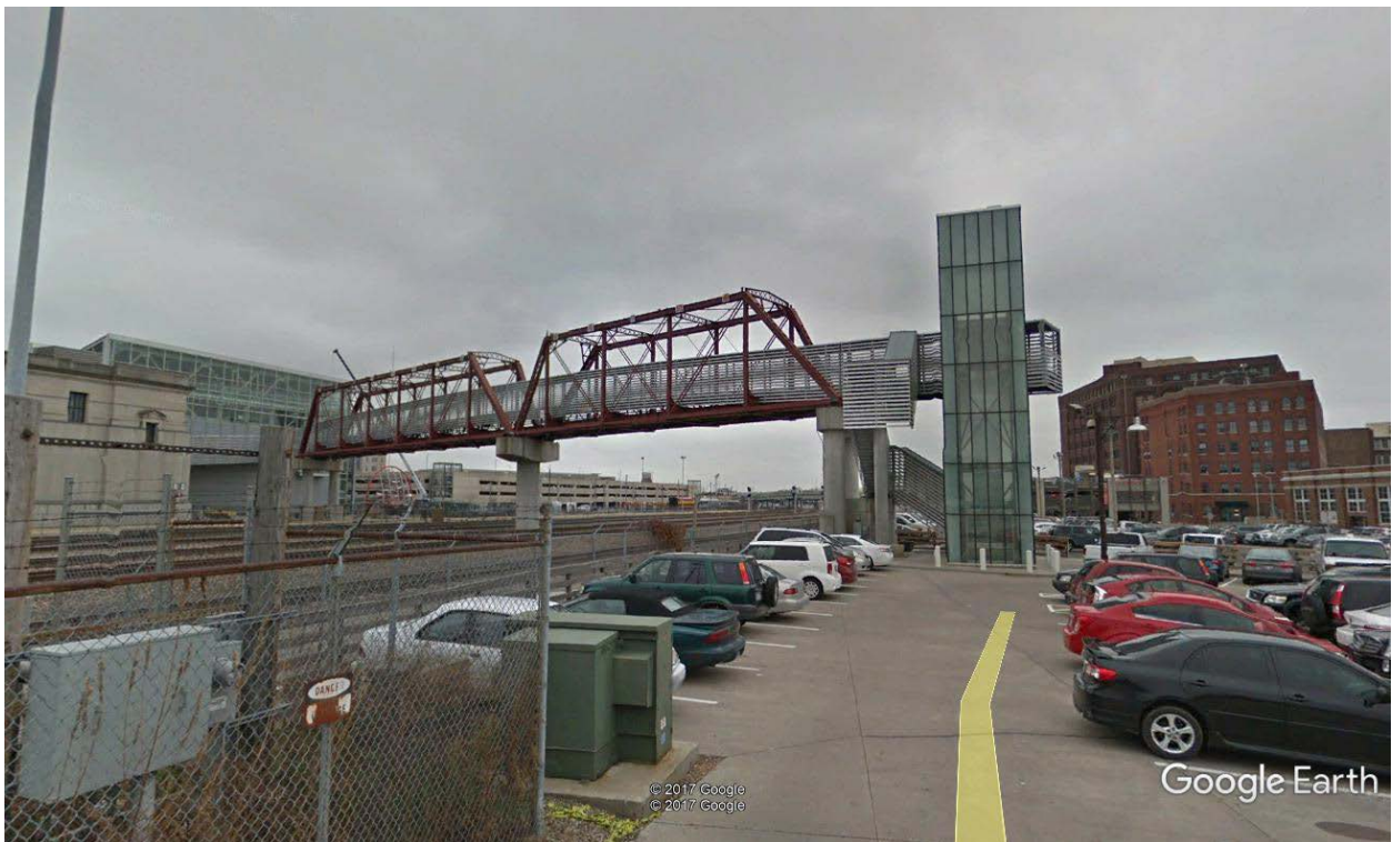
Freight House Pedestrian Foot Bridge, Kansas City, MO
