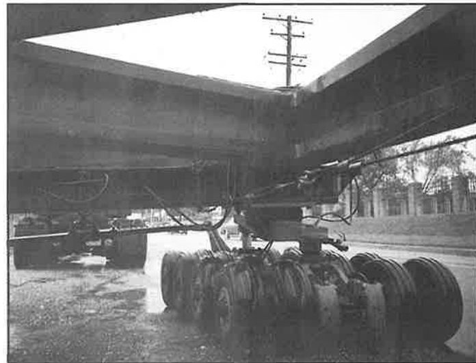
STEEL BEAMS FOR THE CONVENTION CENTER EXPANSION ARRIVED DAILY BY TRUCK.
