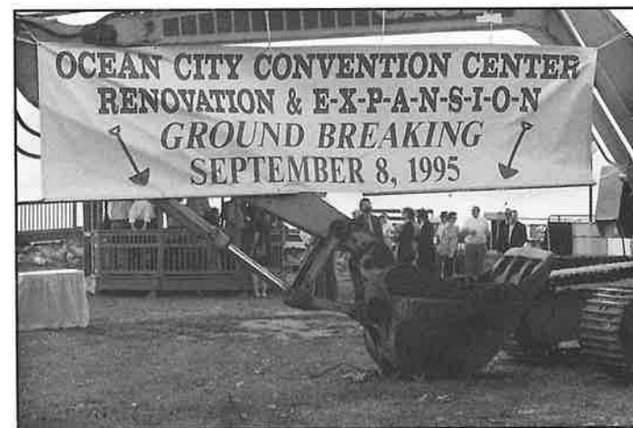
GROUND BREAKING FOR THE OCEAN CITY CONVENTION CENTER IN SEPTEMBER.
