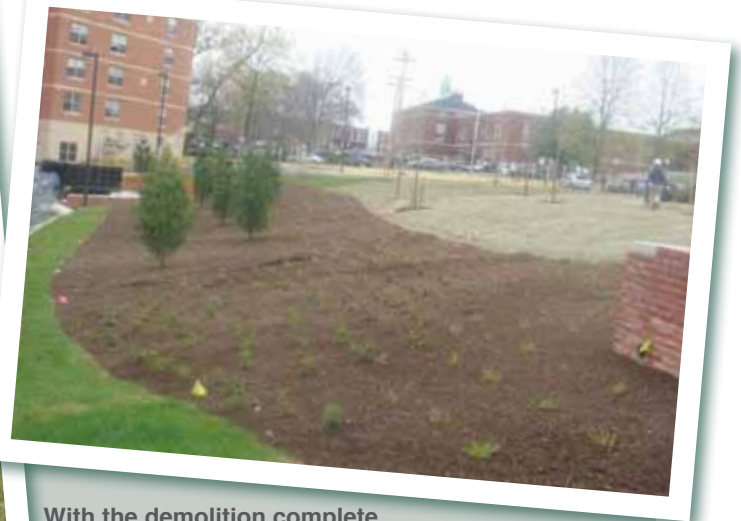
With the demolition complete, environmentally-sensitive landscaping was installed in May to define the campus quad. Project was completed on time, on budget.
