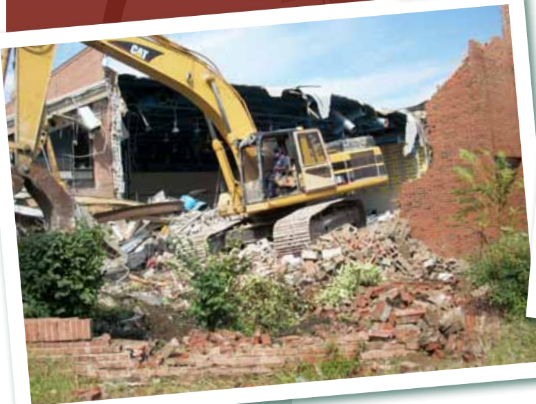
The old Coppin Center was demolished in 2011.
