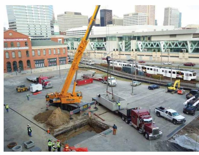
As part of the lot improvements for Pit Row at Camden Yards, the Stadium Authority installed a 7000 gallon underground reservoir to collect rain from the Warehouse roof. This stormwater management device will be pumped for irrigation and power washing, significantly reducing potable water use.
